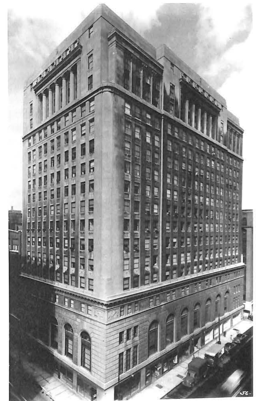
The Chicago Mercantile Exchange building, at Franklin and Washington Streets in Chicago's Loop, was purchased by Material Service Corporation and became its new home in 1948. Price was $2.5 million. It enabled MSC and its subsidiaries to join together in a single office building. Photo taken in 1950.
